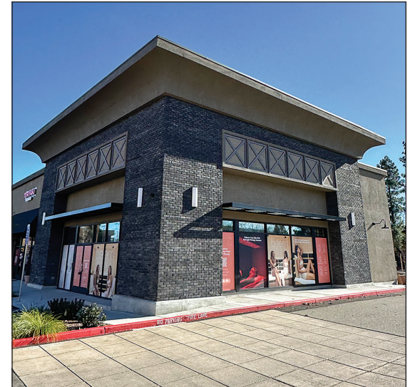
Expected to open in May 2025 at 6455 Owens Drive in Pleasanton.
